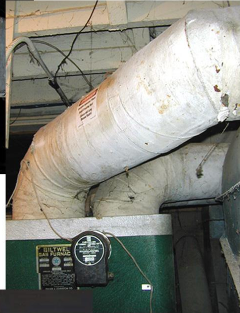
CORRUGATED (ABOVE) AND FLAT (RIGHT) ASBESTOS PAPER ON FURNACE DUCTS
