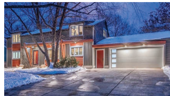
Entire House Under $250,000 Degnan Design-Build-Remodel With Team Members: Coyle Carpet One Floor & Home LLC | Design Electric of Madison, Inc. | R&D Drywall, Inc. | Goliath Tech
